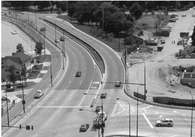
The renovated intersection at Lake Shore Drive and 55th Street now features an underpass for pedestrian and cyclists to access the lakefront.
