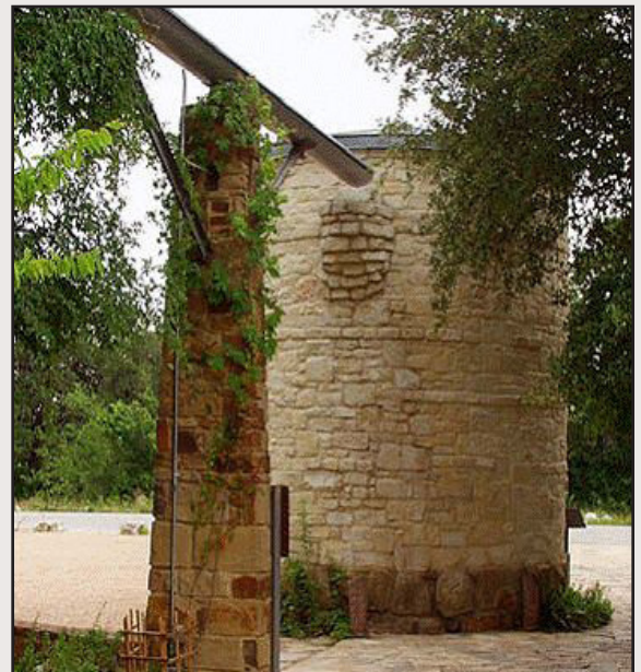
This rainwater harvesting cistern was built in 1995, at the Lady Bird Johnson Wildflower Center in Austin, Texas.
