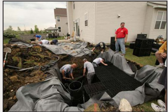
Aquascape employees installing a 1,000 gallon rainwater harvesting system at a home in Oswego, Ill. This water will be used for outdoor irrigation but its not currently tapped for non-potable uses such as flushing toilets.
