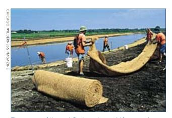
The restoration of Nippersink Creek provides a model for re-meandering, streambank stabilization, and use of native vegetation buffer strips to improve water quality and restore habitat.
